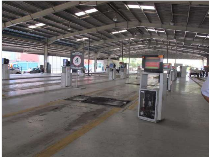
Figure 3 Inspection lane, PUSPAKOM Kota Kinabalu
